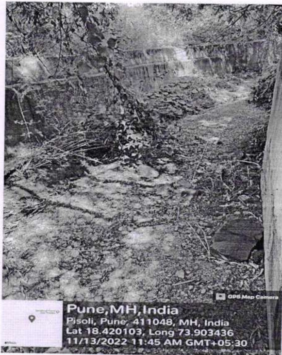
RCC Channel to divert the rain/storm water into water bodies and slow down the flow of water by gradual slope
