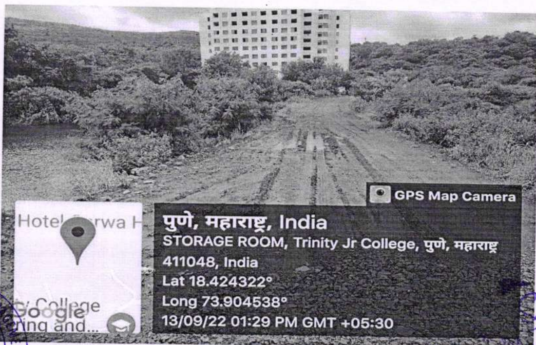
Earthen bunds constructed to create the water bodies
